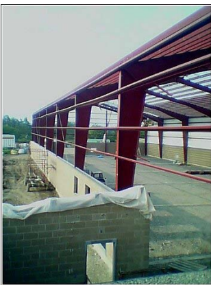
St. Mary's High School project in progress
